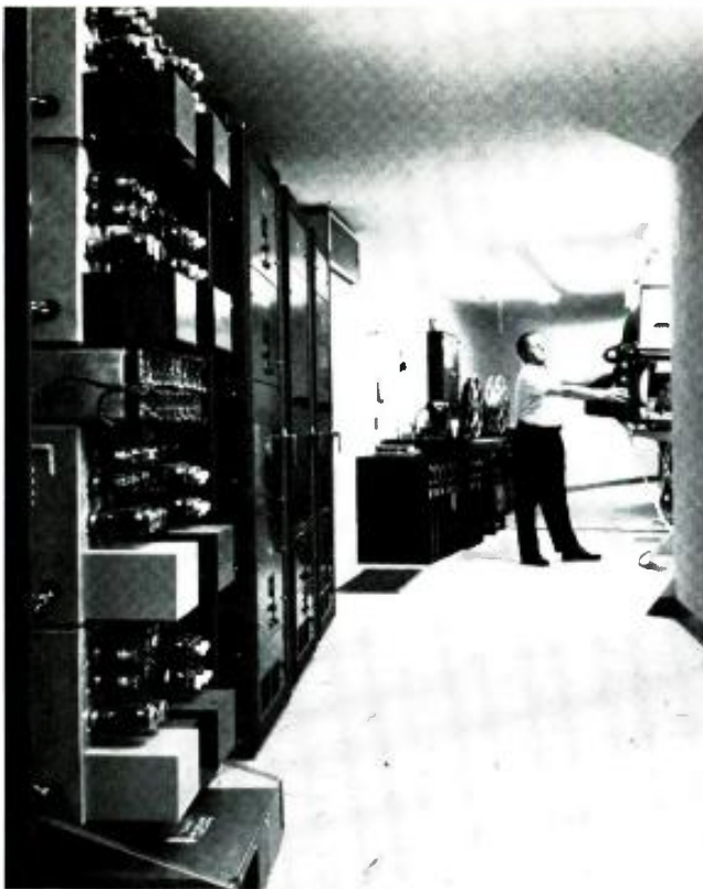
Figure 1. The Century 21 theater in San Jose, California features four racks of a six-channel magnetic theater sound system. This installation has the older vacuum-tube model, which has since been replaced by solid-state units.
